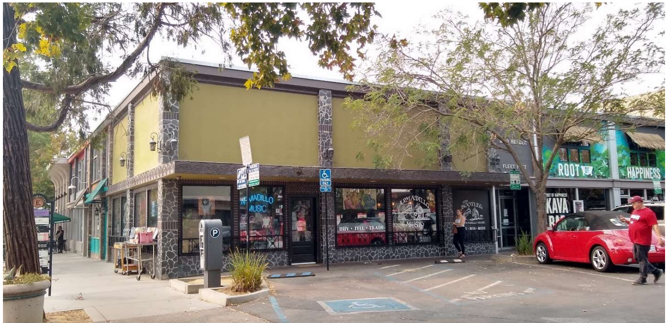
East and north façades, 1963 addition, ESA 2022
