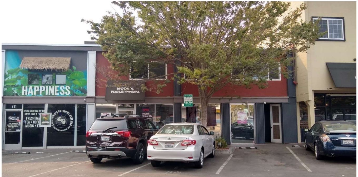
North façade (west end), ESA 2022
